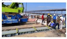
Installation of a TENSA® MODULAR joint on the Sudarshan Setu Bridge
