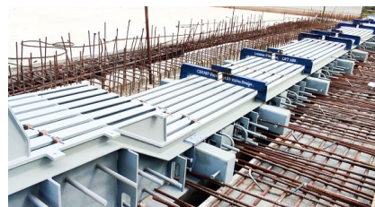
A seven-gap modular joint in its recess
