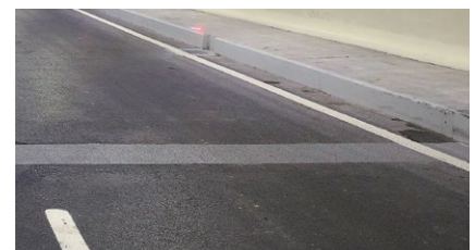
One of the installed TENSA®POLYFLEX® joints
