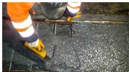
Casting of a TENSA®POLYFLEX® Advanced PU joint
